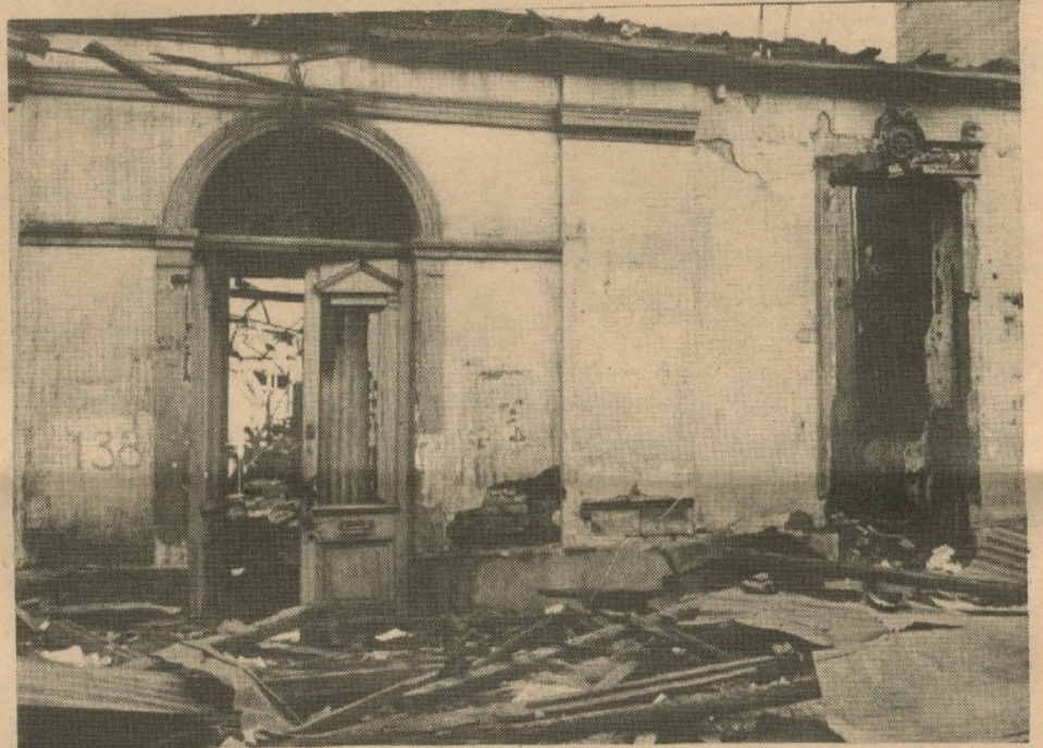
Bombed out headquarters of Socialist Workers Party was one of hundreds of buildings destroyed during the September, 1973, coup in Chile.
